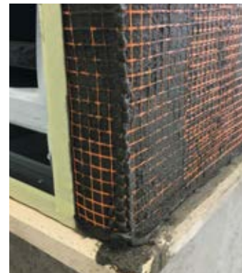
Application of reinforcement and anti-cracking mesh
