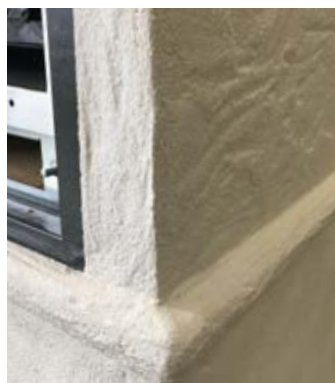
Completion with finish plaster
