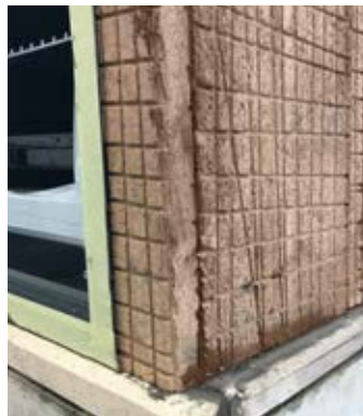
Lining with refractory
